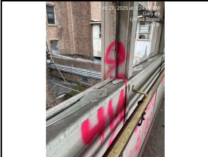
Sample # B-2-41 Window Glaze - Wood Framed Sliding Windows
