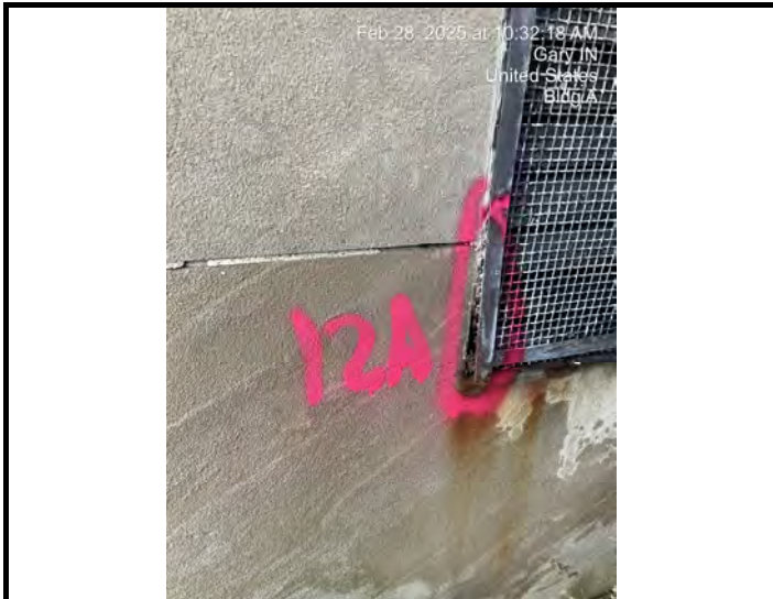
Sample # A-Ext-12 Exterior Caulk-Vent Sealant - On Vents
