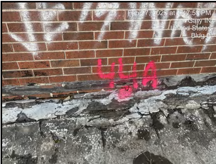
Sample # B-2-44 Roofing Material - Flashing
