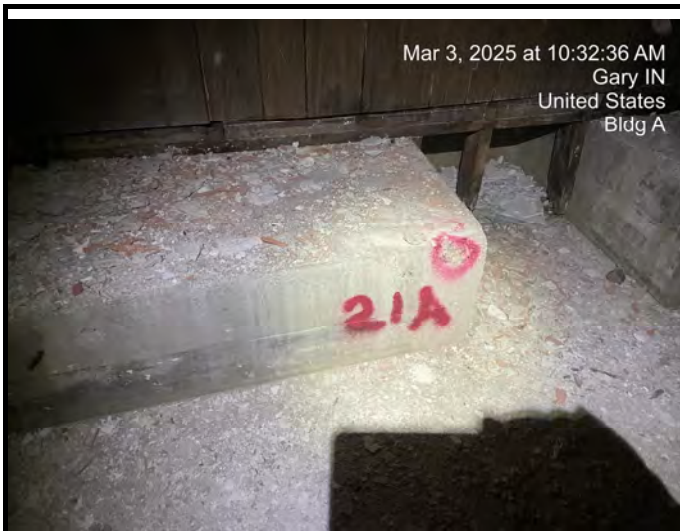
Sample # A-21-Bas Concrete - Walls-Foundation
