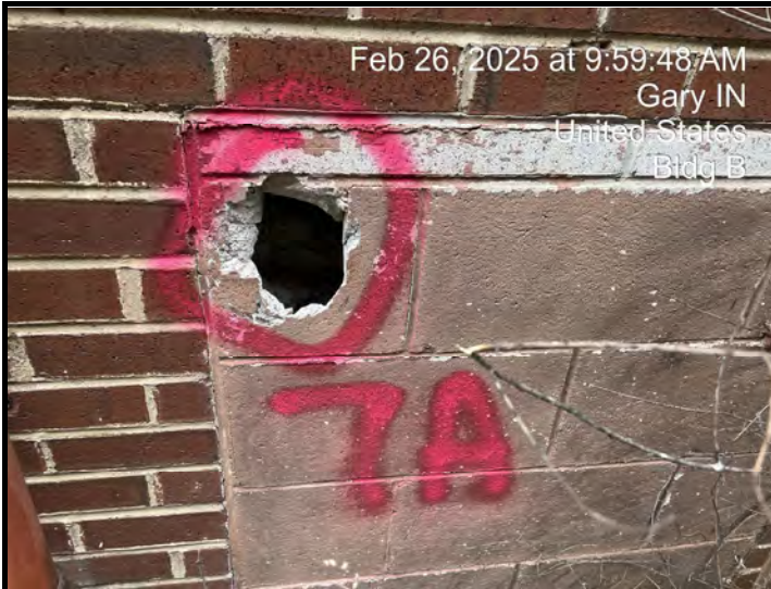
Sample # B-Ext-7 Block Mortar - Patch & Repair of basement windows
