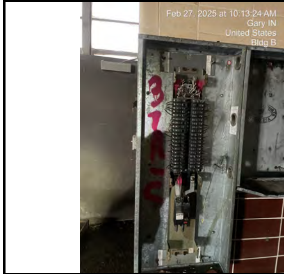
Sample # B-1-37 Insulator - Inside electrical box components
