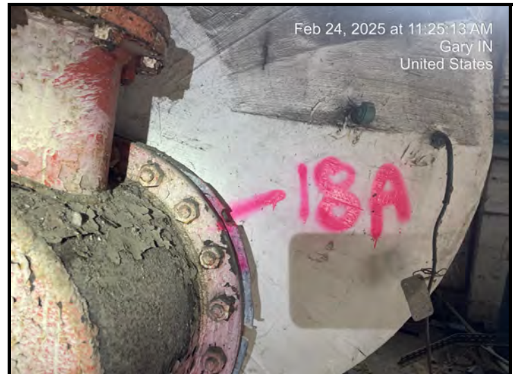
Sample # C-B-18-A-C Gasket Material - Pipe Valves
