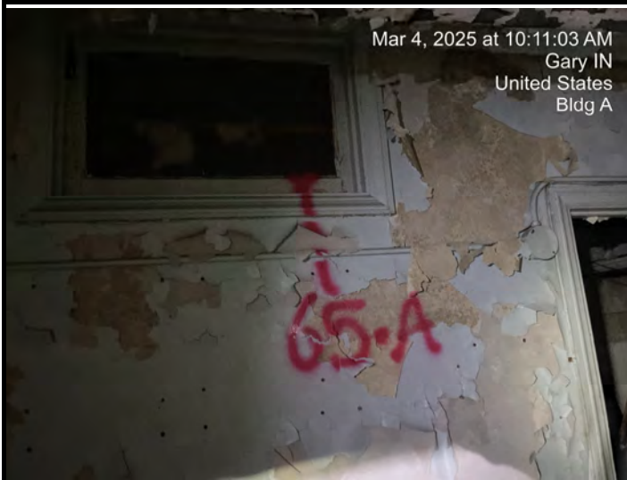
Sample # A-65-Bas Window Glaze - Wood Framed Fixed Windows
