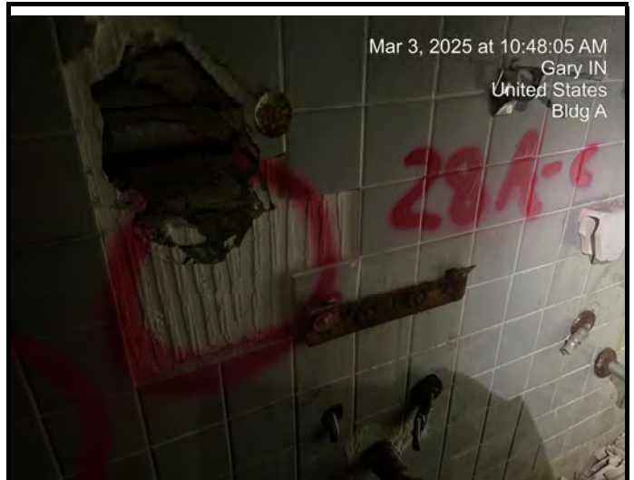
Sample # A-28-Bas Ceramic Tile with Glue - Bathroom Walls
