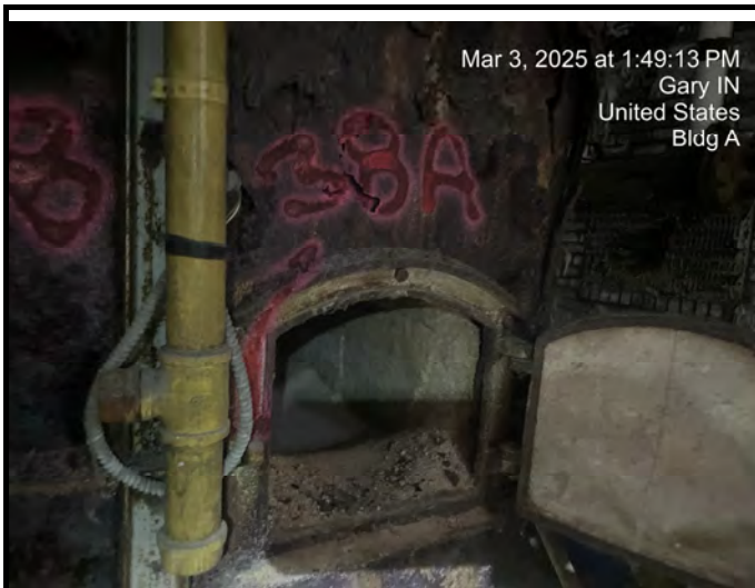
Sample # A-38-Bas Fire Brick - Inside incinerator
