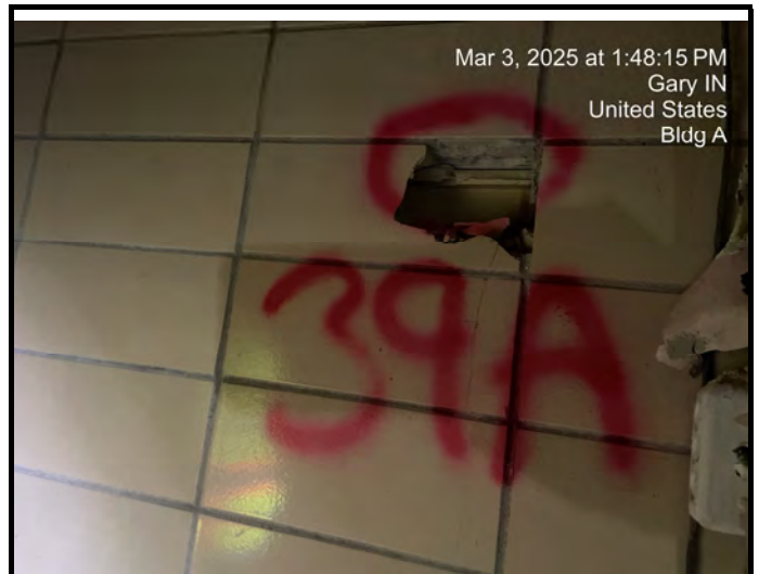
Sample # A-39-Bas Ceramic Tile with Grout - Interior Walls
