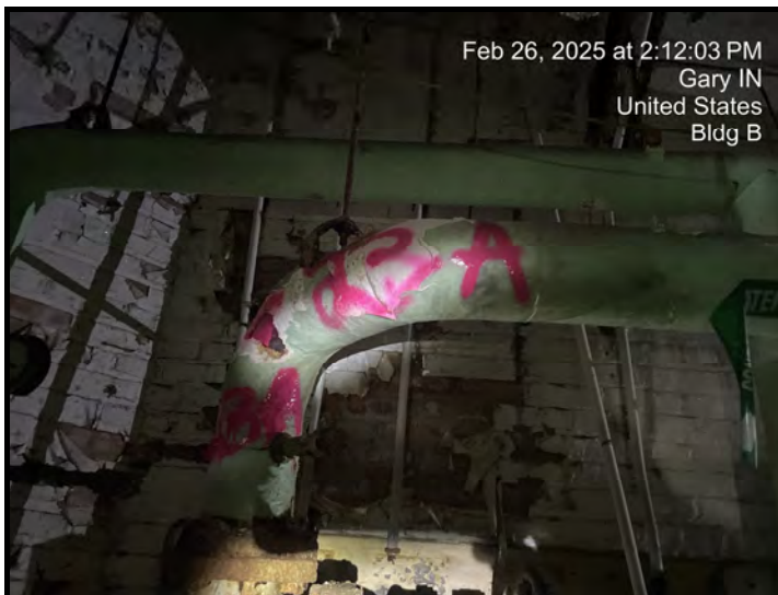
Sample # B-Base-23 Pipe Fitting - 6"-12" Mudded on Fiberglass with Cloth Pipe Insulation
