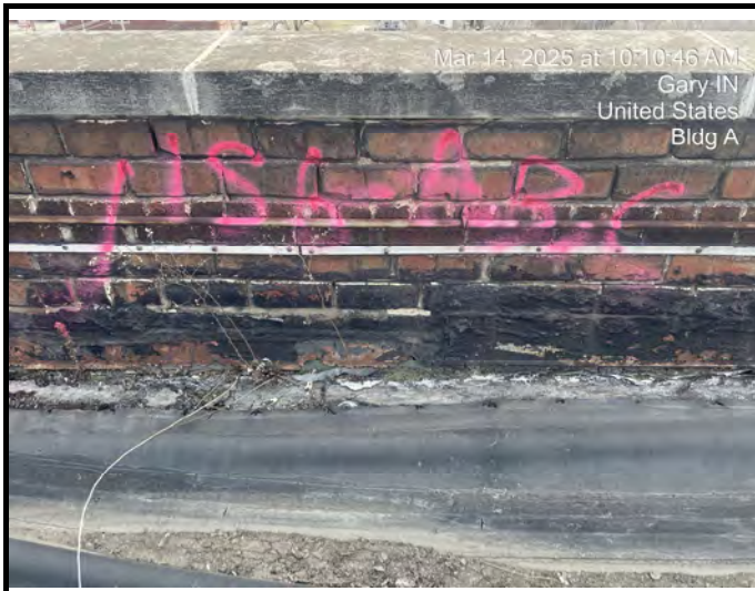
Sample # A-R-156 Roofing Material - Flashing
