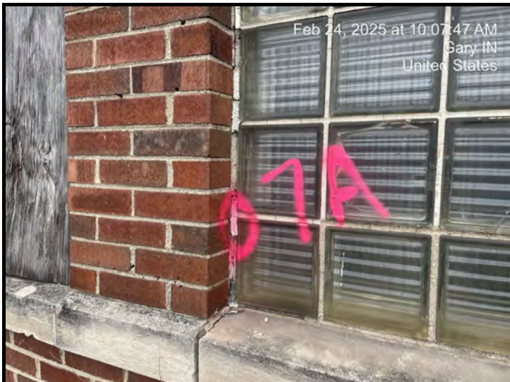
Sample # C-Ext-7-A-C Exterior Caulk - Around Glass Block Windows, Exhaust Window
