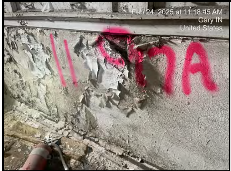
Sample # C-B-17-A-E Plaster - Plaster over Terra- Cotta Walls
