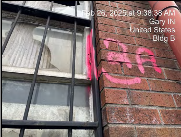
Sample # B-Ext-2 Exterior Caulk - on Brick Siding & Trim, Windows, Doors, Transitions, Seams
