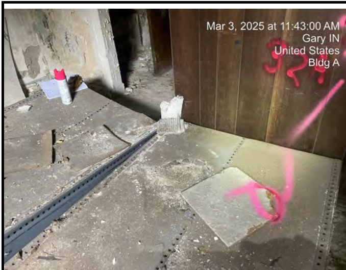
Sample # A-32-Bas Ceiling Tile - 1X1, Smooth with White
