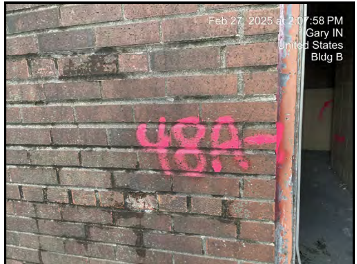
Sample # B-2-48 Exterior Caulk - Door Caulk
