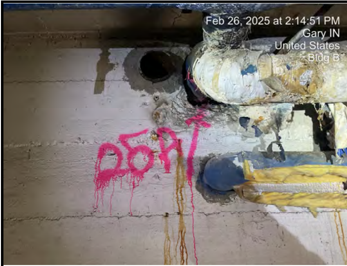
Sample # B-Base-25 Pipe Fitting - 6"-12" O.D. Mudded pipe insulation on fiberglass SRPI
