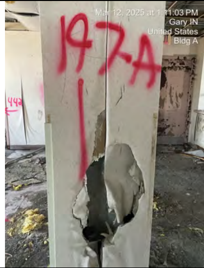
Sample # A-5-147 Wall Sheeting - Layered Paper on walls
