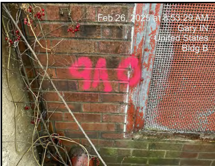
Sample # B-Ext-9 Concrete - Base for electrical cable runs
