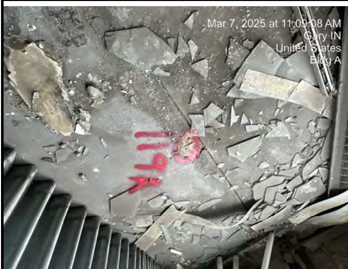
Sample # A-2-119 Flooring - Linoleum with Paper Backing- Blue with mini Squares
