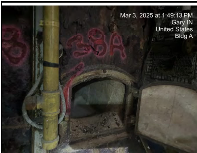
Sample # A-38-Bas Fire Brick - Inside incinerator
