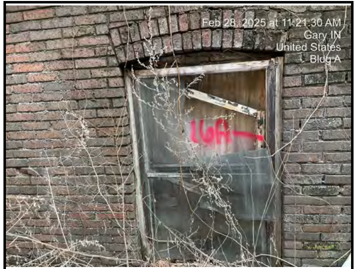
Sample # A-Ext-16 Window Glaze - Wood Framed Sliding Windows
