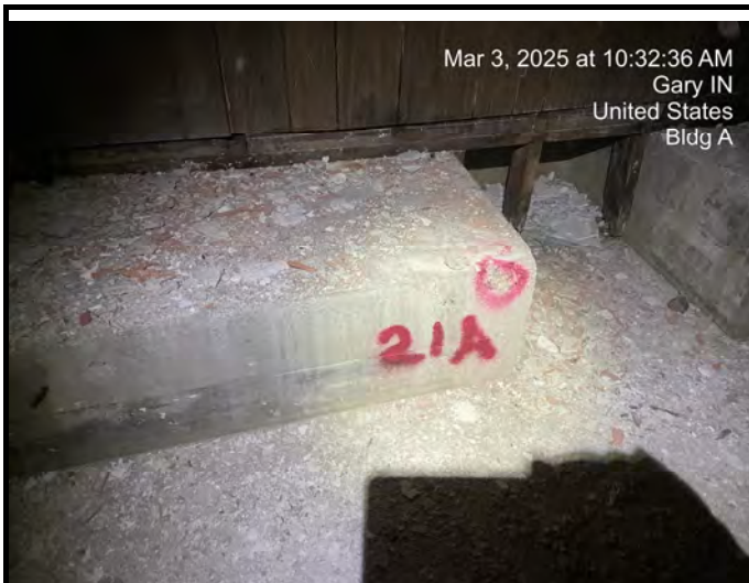
Sample # A-21-Bas Concrete - Walls-Foundation
