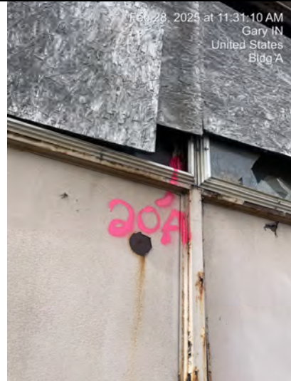
Sample # A-Ext-20 Window Glaze - On Metal Pan Large Windows
