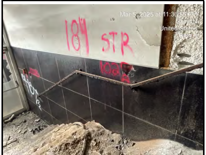
Sample # A-1-102 Marble Grout - Stairway Walls
