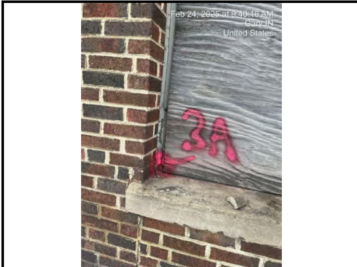
Sample # C-Ext-3-A-C Exterior Caulk - Around wood windows- 1st floor
