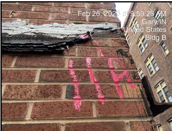
Sample # B-Ext-11 Roofing Material - Flashing
