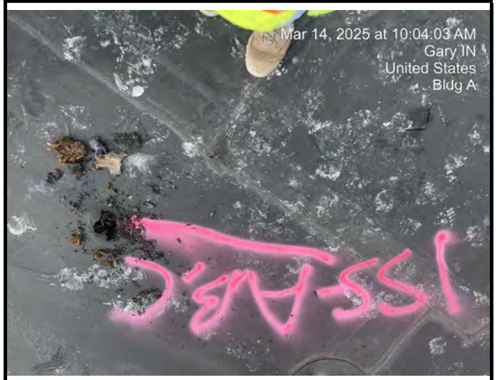
Sample # A-R-155 Roofing Material - Flat Roof Materials
