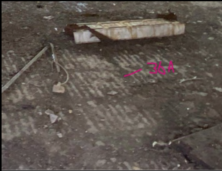
Sample # B-1-36 Flooring - Linoleum with White Paper Backing-TableTop
