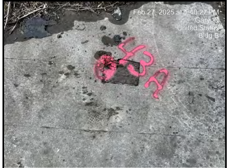
Sample # B-2-43 Roofing Material - Flat Roof Materials
