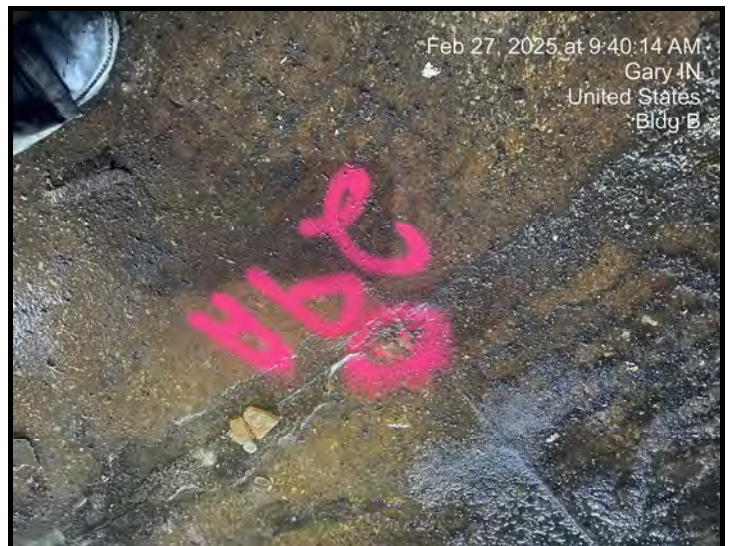
Sample # B-1-29 Flooring - Linoleum with Paper White Backing- Stone pattern
