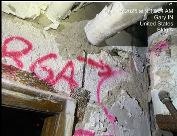
Sample # A-86-Bas Pipe Fitting - 6"-12" O.D. Mudded pipe insulation on Fiberglass SRPI
