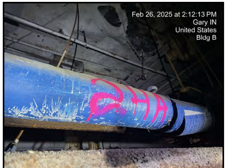
Sample # B-Base-24 Pipe Insulation - 6"-12" O.D fiberglass with cloth SRPI
