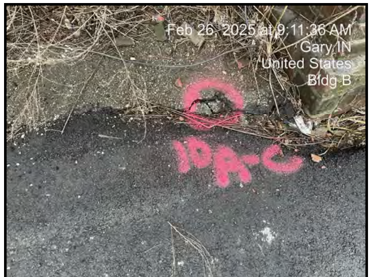
Sample # B-Ext-10 Asphalt Paving - Around structure perimeter
