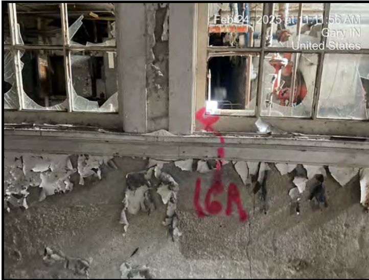
Sample # C-B-16-A-C Window Glaze - Wood Framed Sliding Windows-Interior
